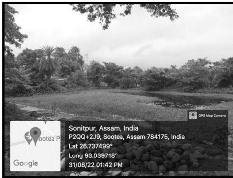
Fig. 7 Photograph showing the Location of proposed construction of Park and Water Sports facilities at Sootea
