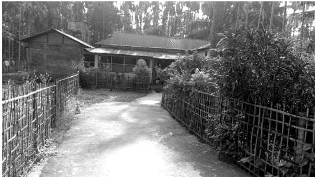
Figure 2.3 Housing Unit at Baithalangso, 2022
