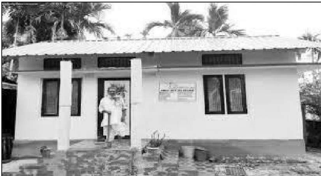
Figure 4.3: A Typical PMAY Unit
