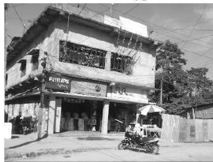
A Typical Commercial and Residential complex
