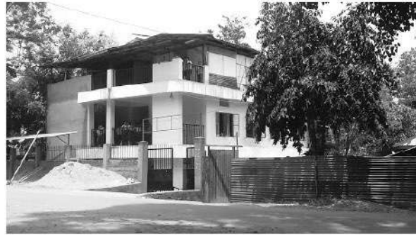
A Pucca house with typical structure
