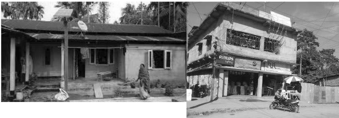
A Pucca house with typical structure
