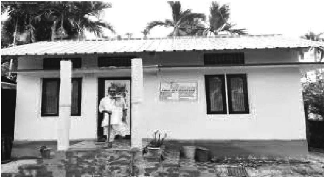
Figure 4.3:A Typical PMAY House in Town
