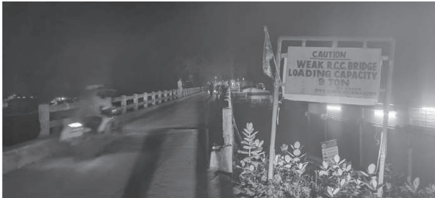
Figure 11: Bridge Connecting Howraghat Town to Nagaon District (Border District)
